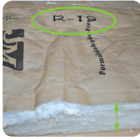
2. Insulation R-value matches work order
