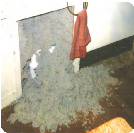
3. Ensure wall integrity is complete (no holes)
