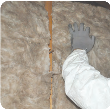
3. Install batts with minimal compression
