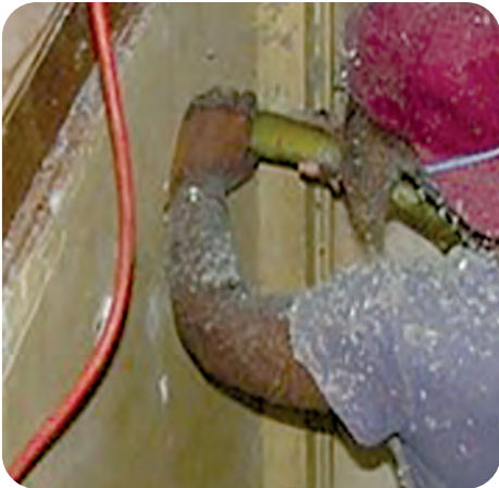
7. Dense pack stairway walls
