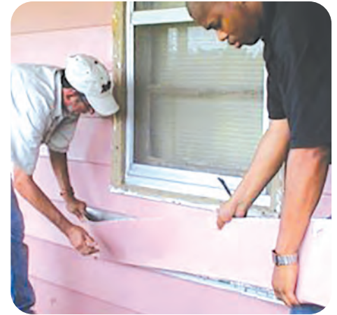
9. Replace and/or repair siding
